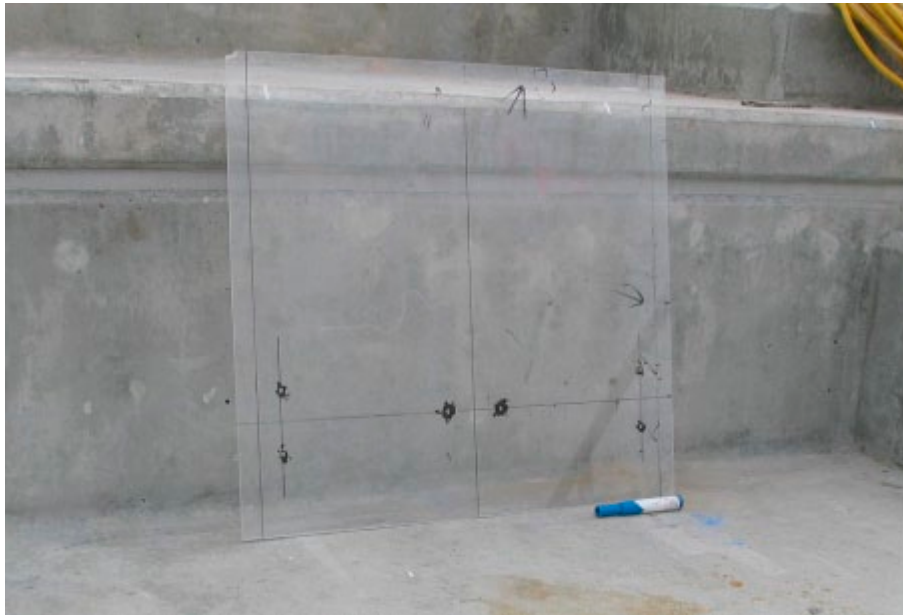
Figure 2: A drill pattern for riser mount standards constructed of acrylic or plexi-glass facilitates installation.
